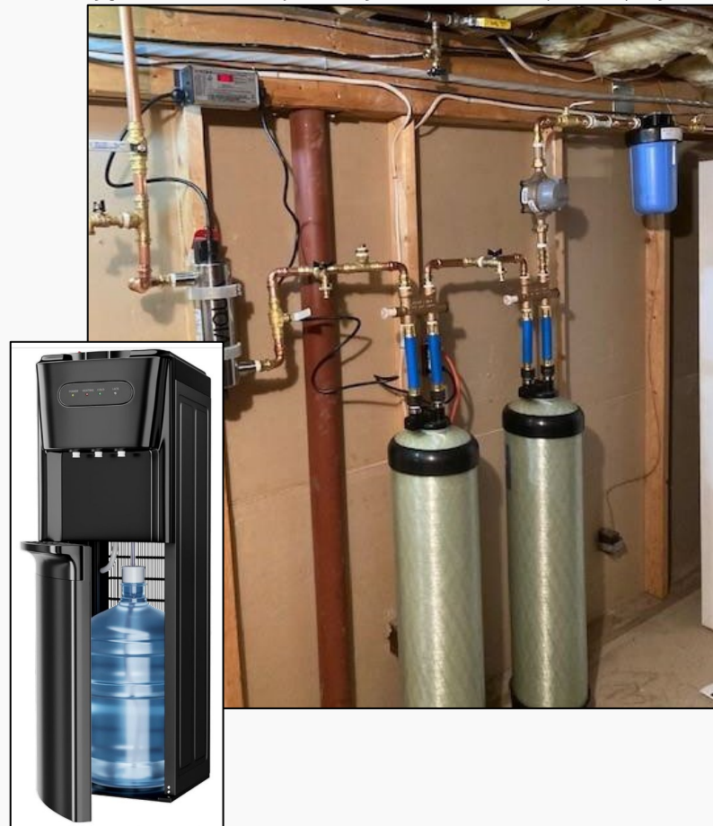
Typical Point-of-Entry Treatment (POET) system
