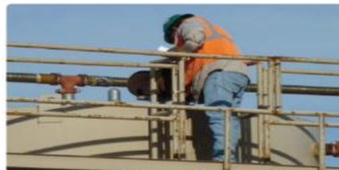
A worker collecting a sample from the open hatch of a production tank. Image: J.D. Danni, OSHA.
